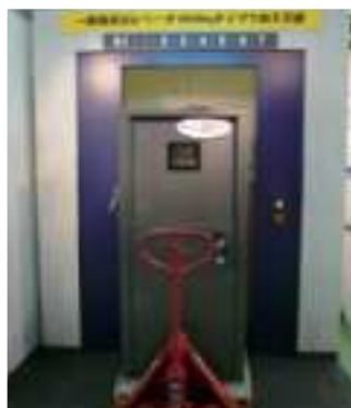
Image picture of Lift instalation.
